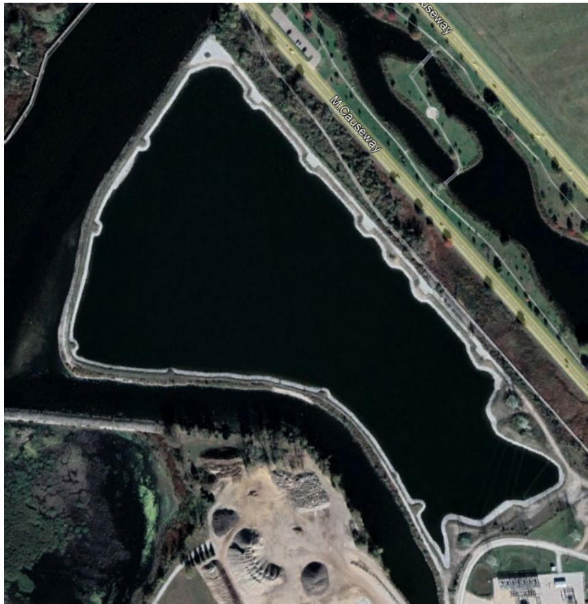
Figure 2. Aerial Image of Impoundment
