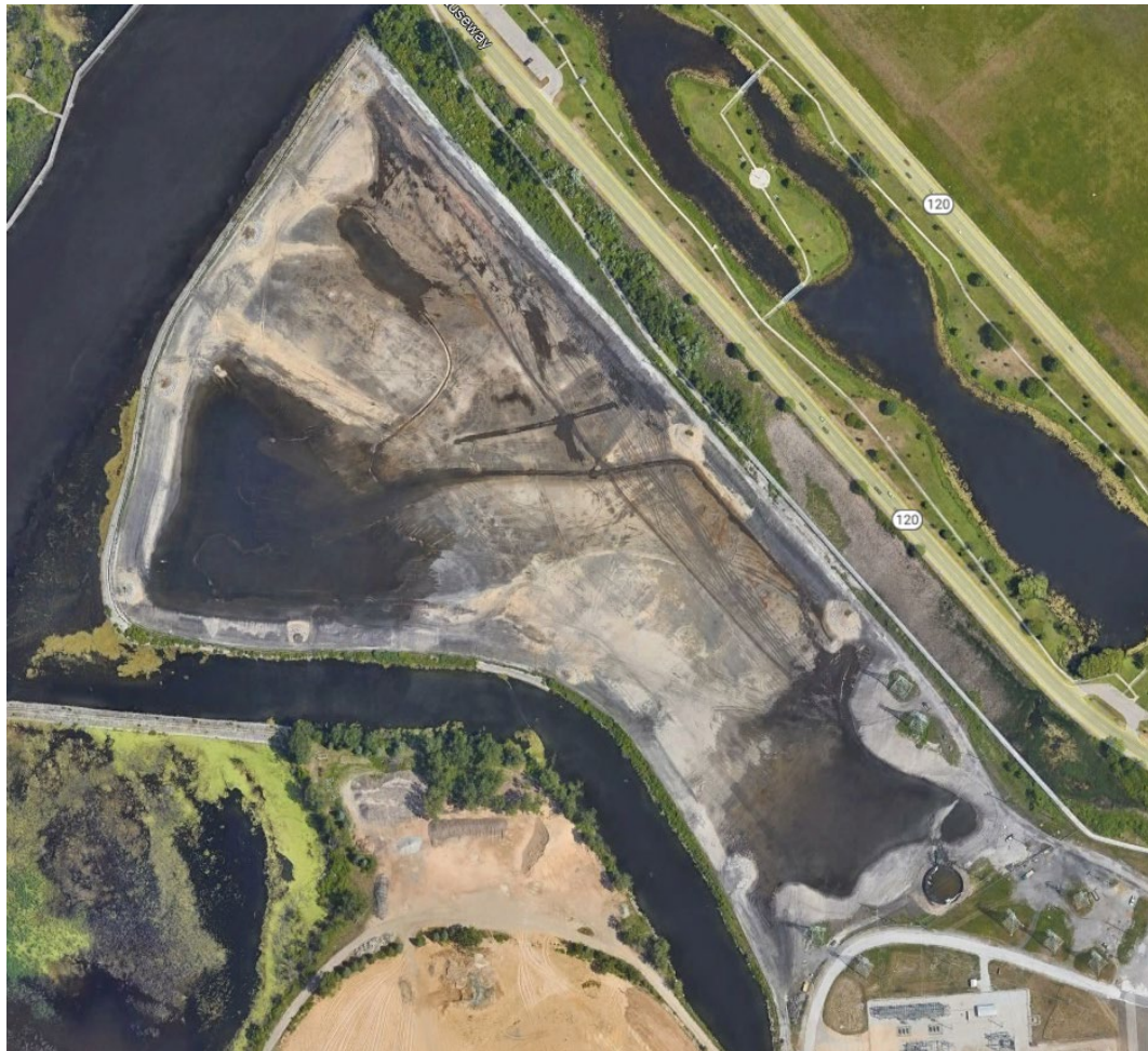
Figure 2. Aerial Image of Impoundment
